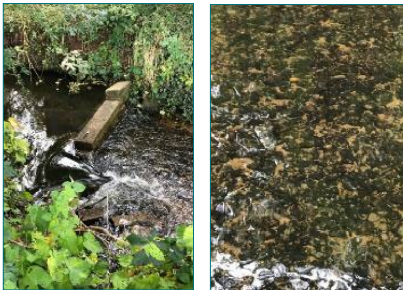
Plate 18.3.15: Weir and Bed Armouring Along the Swannington Beck
